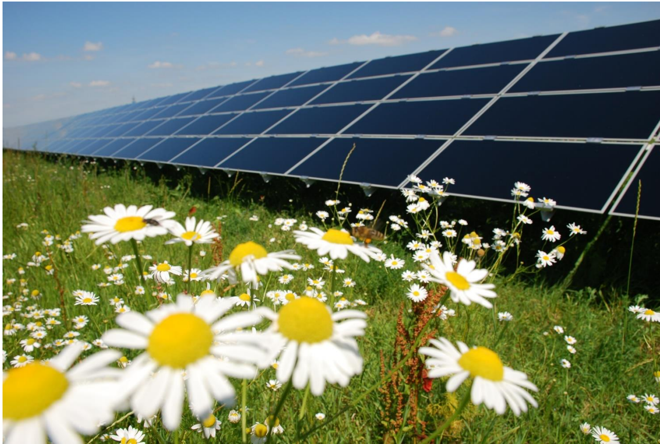
Salmdorf Solar Plant - Germany
